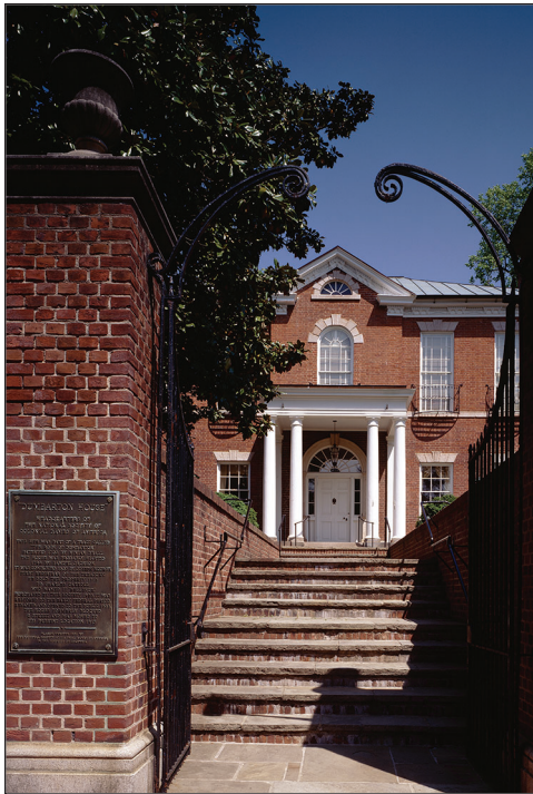
Above: Dumbarton House, built in 1799, is a Federal period house museum in Washington, DC. The NSCDA purchased the house in 1928 and, following restoration, opened it to the public as museum in 1932.
